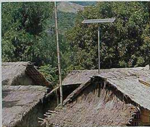
Solar Home Systems in Gregorio del Pilar, Ilocos Sur. The 70Wp system with five lights is the pride of the tobacco farmer's household.
