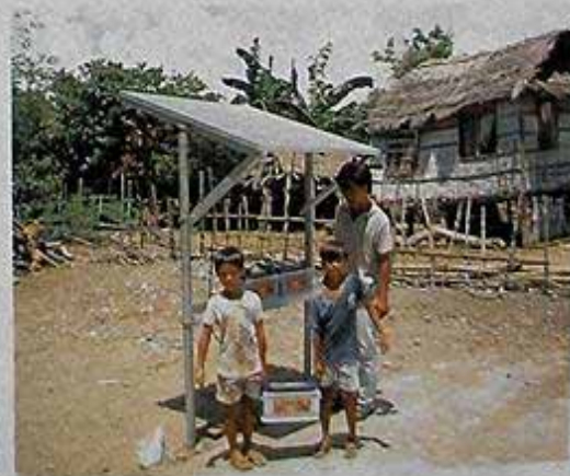
Battery Charging Station in Baccara, Ilocos Norte. The simple 200Wp unit is a neighborhood concept and operates commercially at $1 per battery charge.
